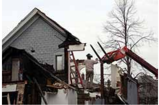
A deconstruction effort in Buffalo by ReUse Buffalo
